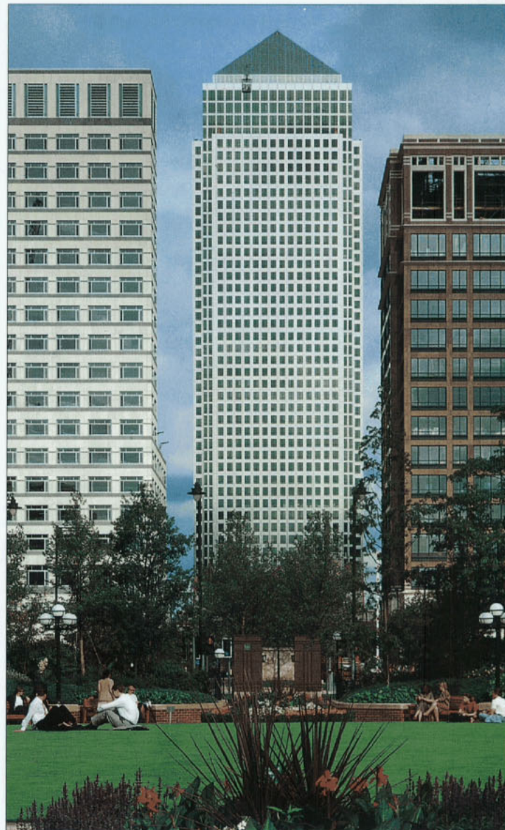
above: Canary Wharf, Infrastructure, London
