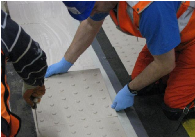
Application of Section 12 Platform Blister
