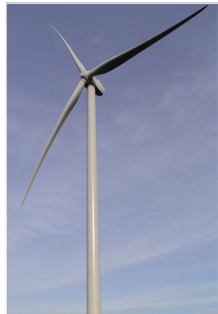
Waterproofing of wind turbines bases on behalf of Merck, Sharp & Dohme Ltd,
